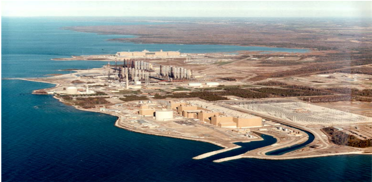
Bruce A & B with Heavy Water Plant
